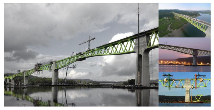
The viaduct over the River Ulla belongs to the new Atlantic stretch of the high speed railway line, in particular, to the stretch between Villagarcía de Arosa and Padrón. The structure of this viaduct consists of a composite deck with a tubular section within which the trains will circulate. This tube is supported by vertical piers and by triangular cells in the area of the river crossing so that the main span length may be increased without increasing the lintel span.
